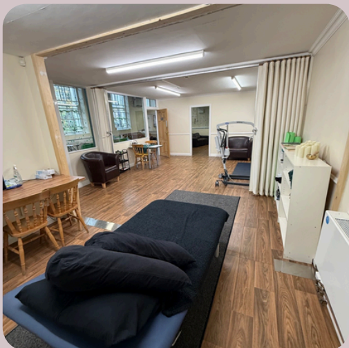
Clare Road renovation
